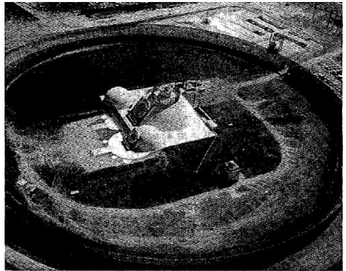
Figure 4 Clutter suppression fence for MAR installation at White Sands [5]
